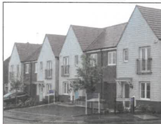
Fig 5.63 Buildings with prominent gable ends creating a strong character (Tilia Place, Dunstable)
